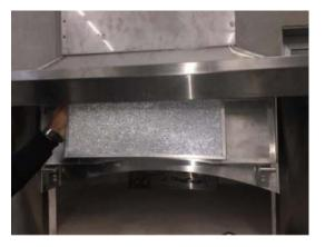
STEP 4: Slide filter panel back up into position inside the exhaust spigot making sure to rest on the centre holding bracket. The angled tabs on the side of the panel will position the panel into the required angled location.
