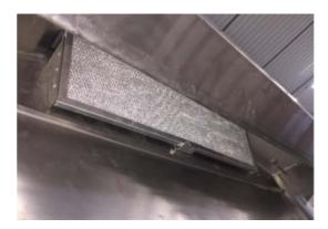
STEP 2: Gently remove the panel by pushing the filter "up" to dislocate the panel from the centre holding bracket.
