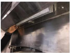
STEP 3: Slide the filter panel down and out of the spigot.
